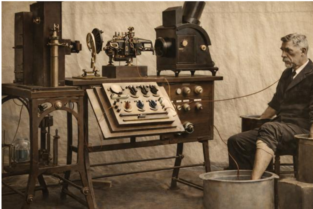
Figure 1. The first electrocardiograph based on the string galvanometer used by Willem Einthoven in the early 20th century (6,7,53).
